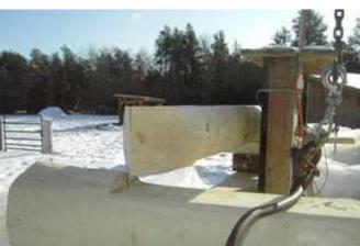
Then set the butting log with the point so that it is setting level onto the log with the natural tail (the passing log) and check to see if the two outer points line up with each other. Sometimes you will have to adjust the angle on one side of the point that you just cut so that they line up especially when the log below has a flare and is wider on one side that the other. Then trace it on the log below and cut it out and fit if necessary.
