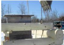
Next I like to match the edges so I trace the log and drawknife the wood off and round it some. You can also use a sander / grinder or chainsaw. I like to finish it up with the drawknife because it closes the pores in the wood and the stain matches better.
