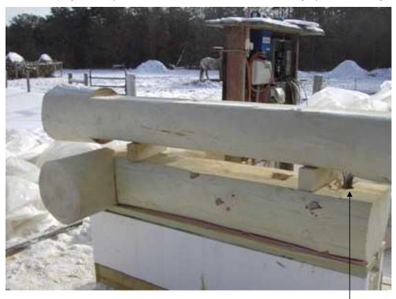
Notice that the electrical wires get a hole drilled or cut up through the middle of the log.
