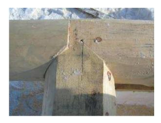
Next set the next passing log with the natural tail up on equal size blocks about 3 or 4 inches high. Be sure and line it up right where you want it and remember to hold the tail in slightly like the first log.
