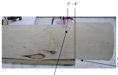
The notch on the bottom side was extended two inches past the foundation so that false stone can tuck under it.
