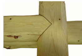
Top view of the V-cuts
