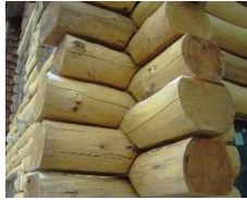
Custom Saddle notch on-site only
