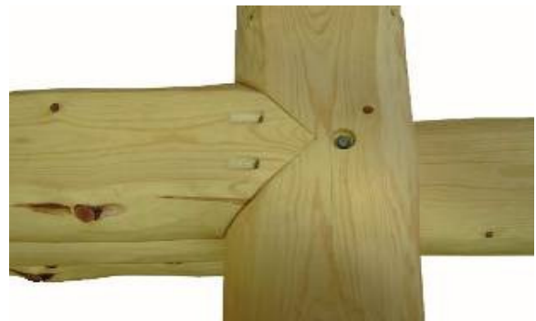
Top view of butt and pass notch
