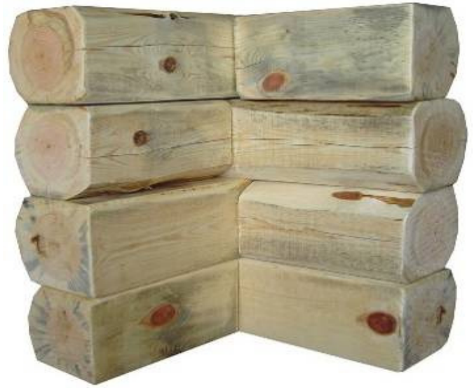
Inside view with wane on the corners
