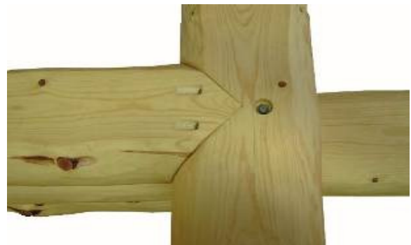
Top view of butt and pass notch
