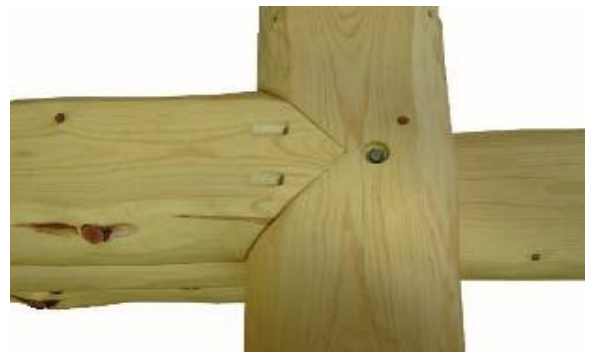
Top view of butt and pass notch
